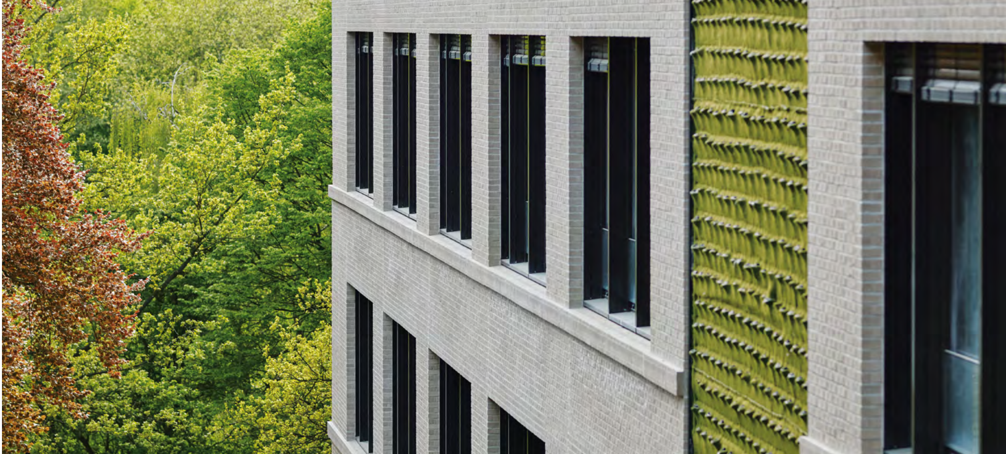
FLOW in Hamburg sets new standards in terms of sustainability and vibrant urban architecture: Vertical greening brings color to the city and ensures a pleasant microclimate – the plant pockets of an innovative fleece substrate system visible here allow facade greening without direct contact with the building structure.
